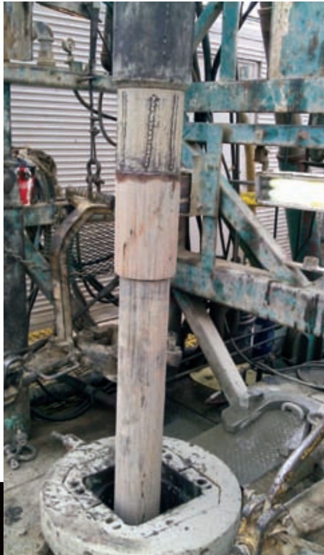
View of a desalter well being drilled.
